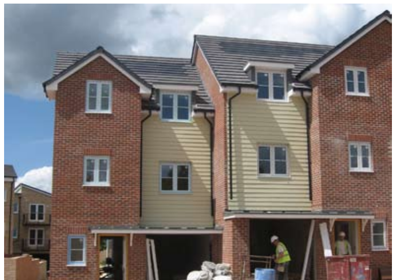
The Linden Homes development in Hampshire, a job by Avonside Roofing following completion of the Solarcentury C21 training course.
